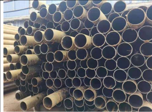
Visual inspection (rusted on the outside and inside surface)
